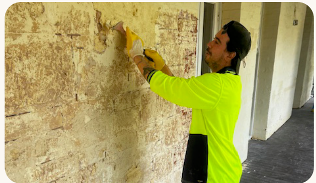
Pic 1: A worker carefully chips away on cement rendered walls that have for decades covered the beautiful original ones built over 120 years ago.
