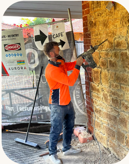
Step 2: Drill out decayed mortar between bricks
