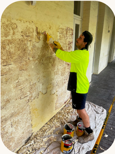
Step 1: Remove cement render coating
