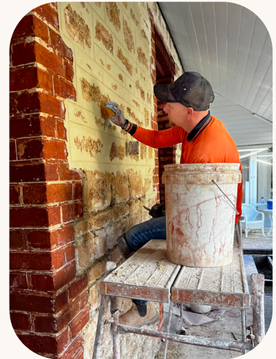
Step 3: Apply new mortar between bricks
